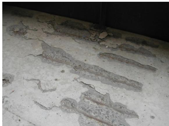
*Figure 2: Surface Spalling*
